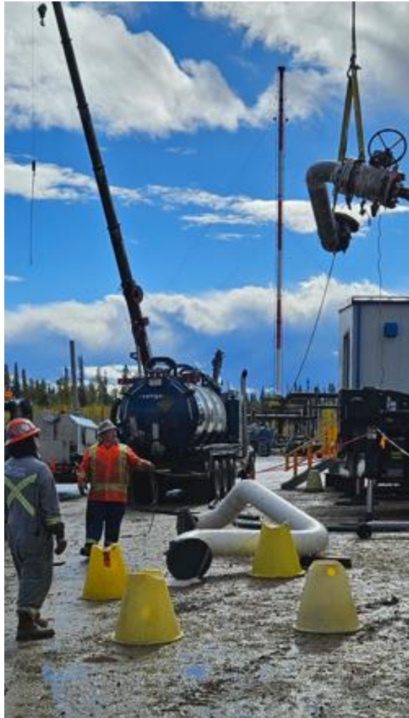
Demonstrating: Tag line use, spotter/communication with crane/clear line of sight with operator/rigging.
